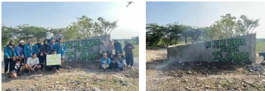
Gambar 8. Pekerjaan Finishing Dinding TPSS
